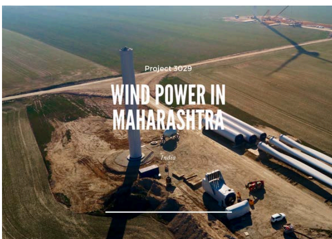
Project 3029: Wind Power in Maharashtra
